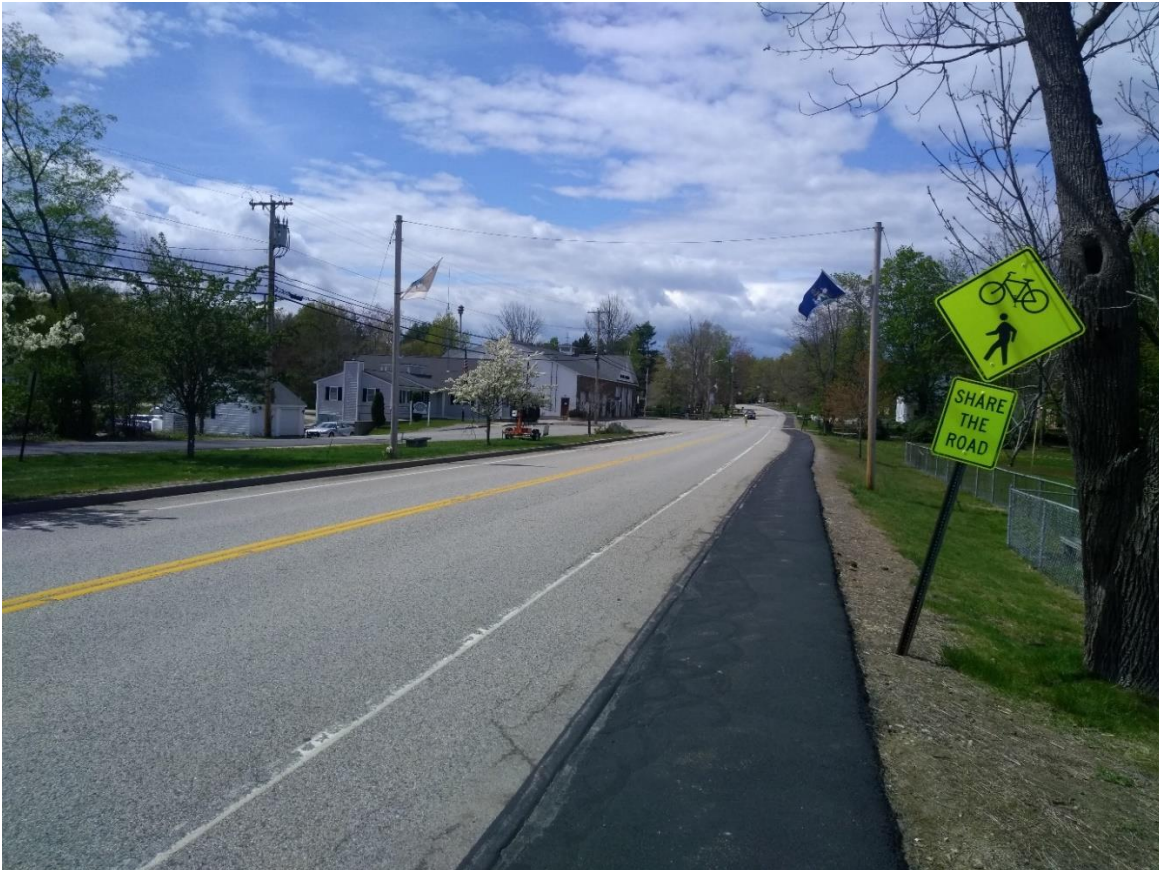
Figure 3. The existing sidewalk, wide shoulder, and “Share the Road” signage on State Rd.
