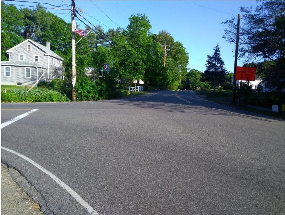
Figure 27. Beech Rd. at its intersection with State Rd. (Farmer's Corner), looking southeast. When combined, the priority projects in this report would add sidewalks, paved shoulders, and marked crosswalks at this intersection.
