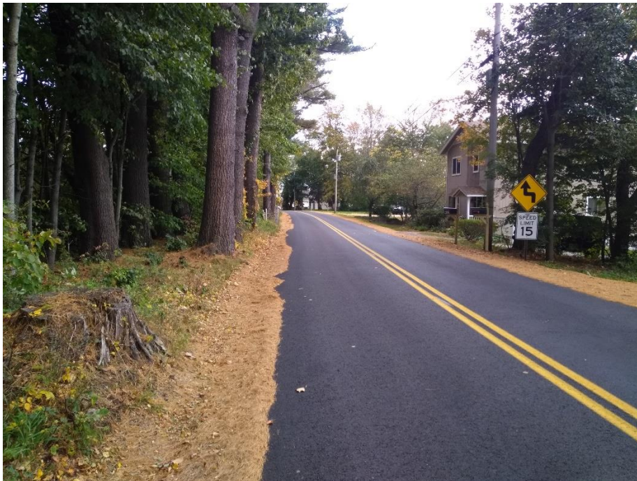
Figure 36. Pine needles effectively narrowing the roadway on River Rd., which already has a low posted speed limit (15 mph). The pines are offering a glimpse of one of the traffic calming elements (roadside narrowing) of a yield roadway concept. Another would be the removal of the double yellow centerline.
