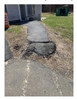
Works for removing and prepping for the sidewalk replacement on the side of Town Hall which was identified by our P&C insurance carrier as an eminent and serious hazard.
