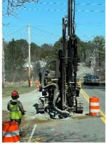
The work has begun on the Water and Sewer Extension Project. Most of the work being performed presently is on Beech Road and State Road as Defelice the contractor on the project is presently drilling test holes to make a ledge determination for the area. As most residents know there is a ton of rock looming just below the surface, some outcroppings not even below the surface.
