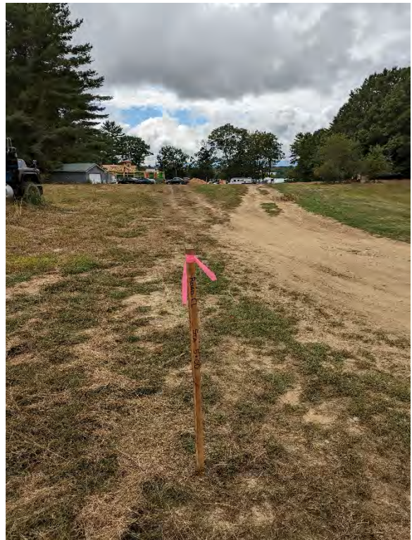
Sta: 5+00 looking west towards river
