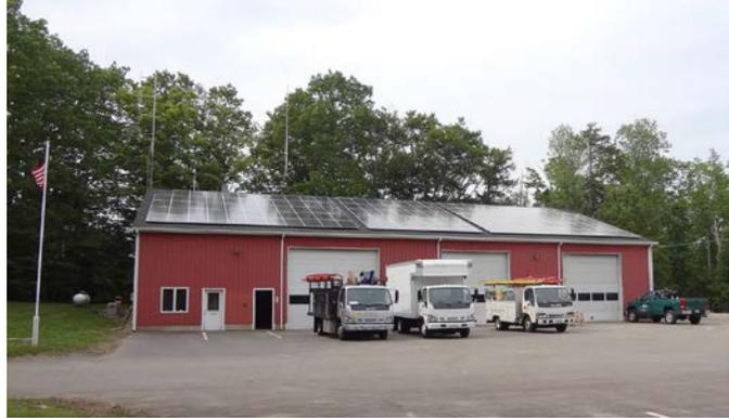
This system was commissioned on June 28, 2013. It is a 41.25 kW grid-tied photovoltaic solar energy array. It consists of 165 Canadian Solar 250-watt panels, 4 inverters, a data logger and remote monitoring system. As of December 31, 2016 it has produced 138,800 kWh of zero-emission solar power.
