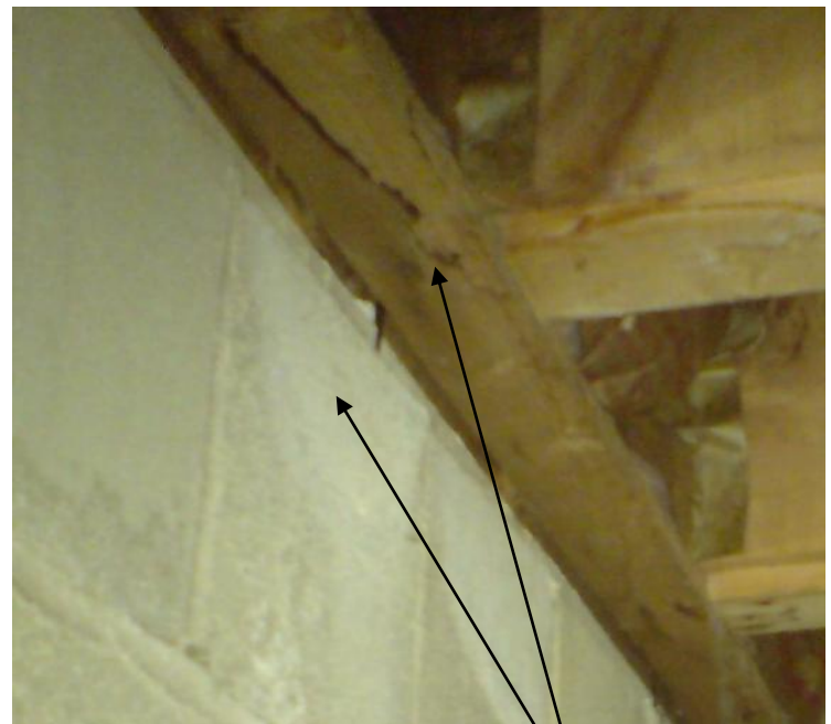
View of band joist showing cold (blue) air infiltration. Note signs of moisture on wall & strapping, likely caused by condensation
