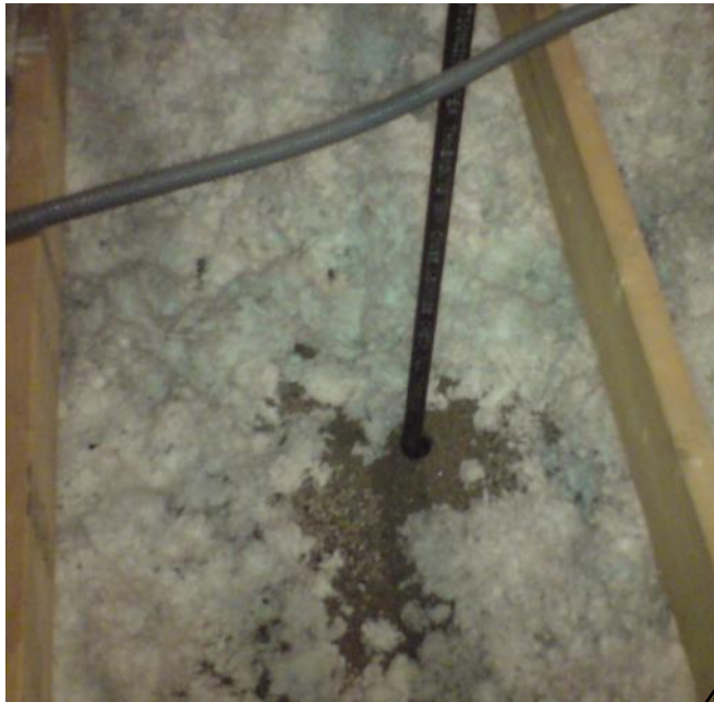
View of area where insulation has been pushed aside showing heat loss (yellow) through thin insulation & around pipe
